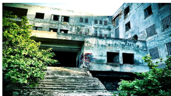
Figure 2. The renovated entrance of the Xenia Hotel with the stairs added to create a lobby.
